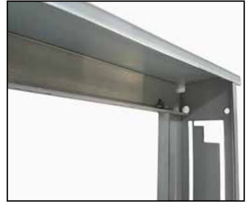
Detailed corner assembly of counterframes B - A.
